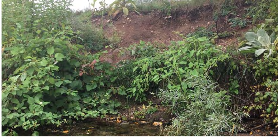
Major slumping in Kensington Metropark.
