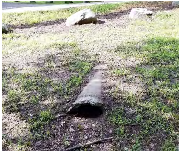
Proportion of outfalls in each condition category. Right: Blocked outfall in failing condition in Kensington Metropark.
