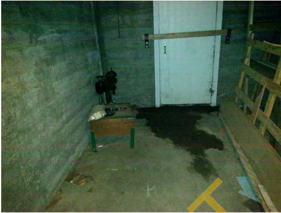
Photograph #3: Near Middle of Newer Basement Addition
