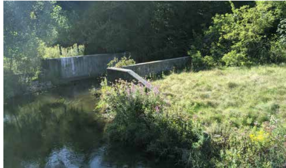
Existing Bridge abutment over Ore Creek
