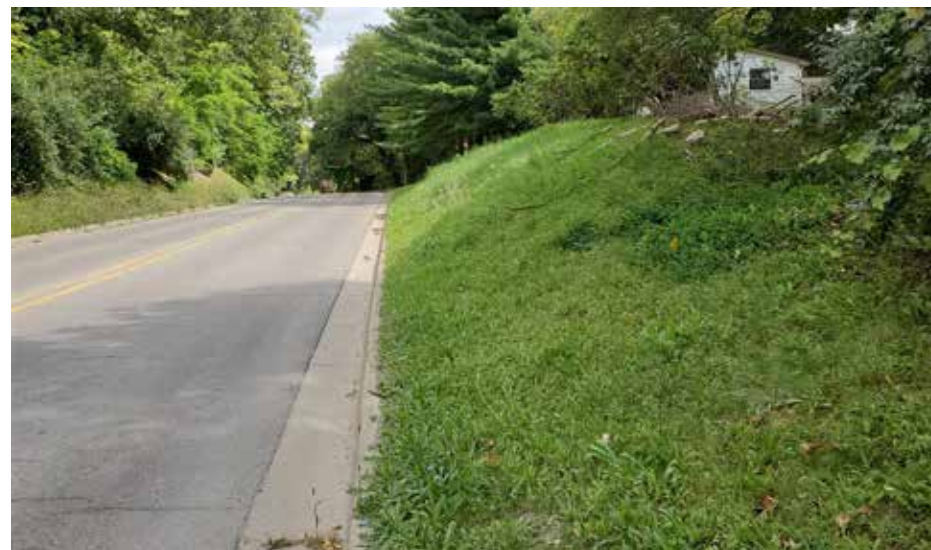
Steep elevation along Maltby Rd
