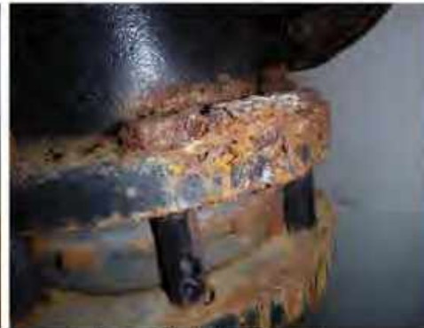
Image 38: Valve Corrosion
