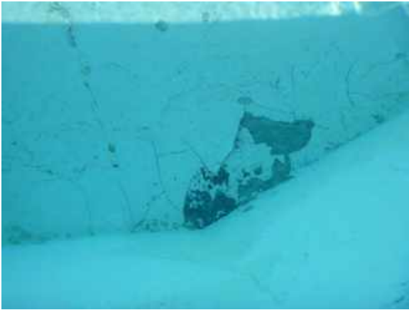
Pool cracking
