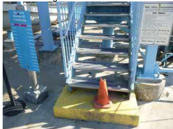
Slide entrance and caution cone
