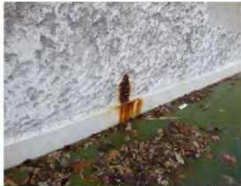
Image 4: Corrosion Bleed-Through
