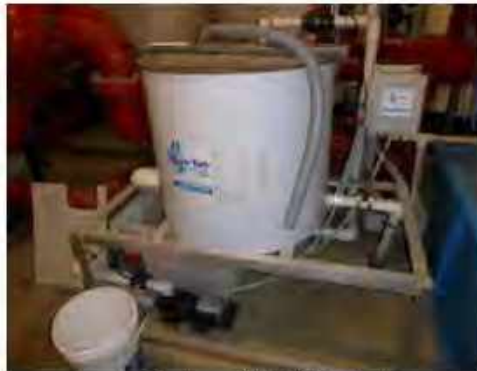
Image 67: Accu-Tab Chlorinator
