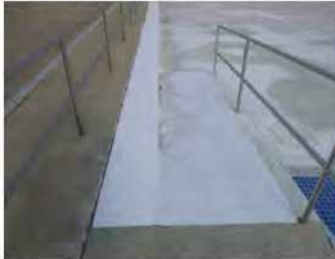
Image 20: Ramp Entry and Barrier Railing
