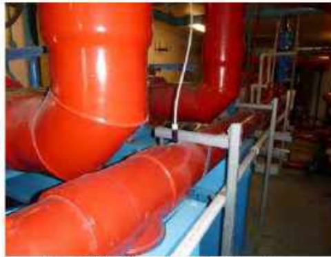
Image 72: Chemical Injection Tap
