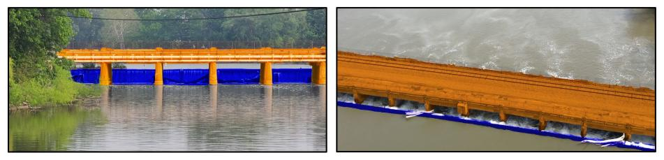
Caption: The Flat Rock Dam is largely a spillway that is submerged under the Huron River. The concrete structure that you see highlighted in orange in these photographs is a bridge owned by CN Rail. The areas highlighted in blue are the dam structure submerged under the river.
