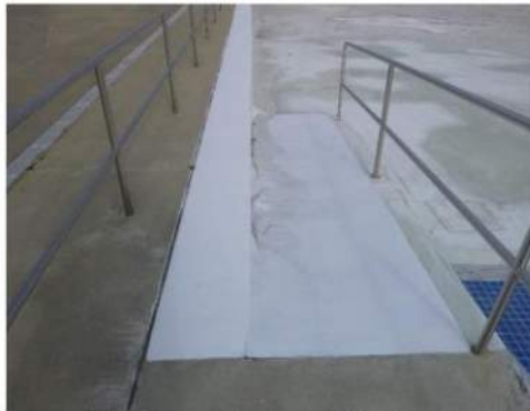
Image 20: Ramp Entry and Barrier Railing
