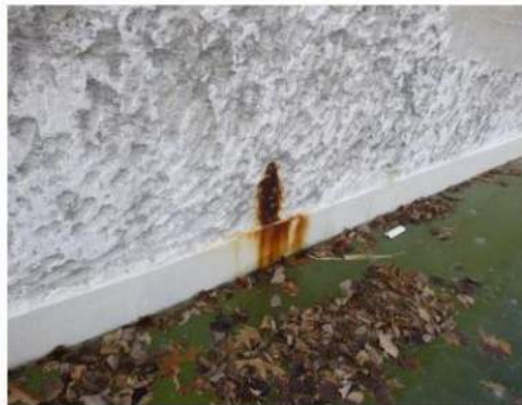
Image 4: Corrosion Bleed-Through
