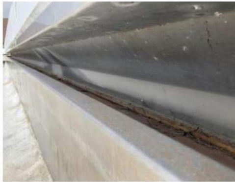
Image 14: Interior Gutter Channel Profile
