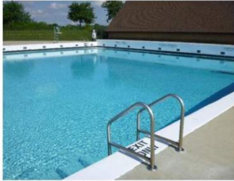
Image 17: Gutter Operating at Surge Weir Elevation
