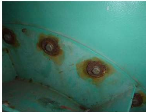
Image 85: Corroded Fasteners
