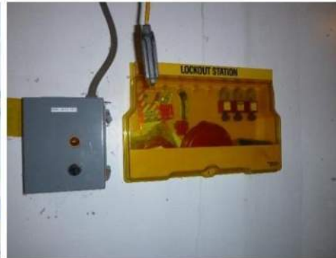
Image 87: Water Level Control Panel
