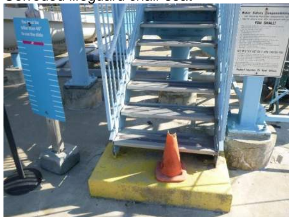
Slide entrance and caution cone
