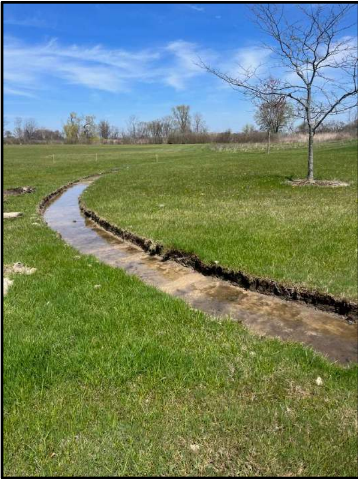
Pictures: Green Infrastructure installation, April 29 th at Lake Erie Metropark
