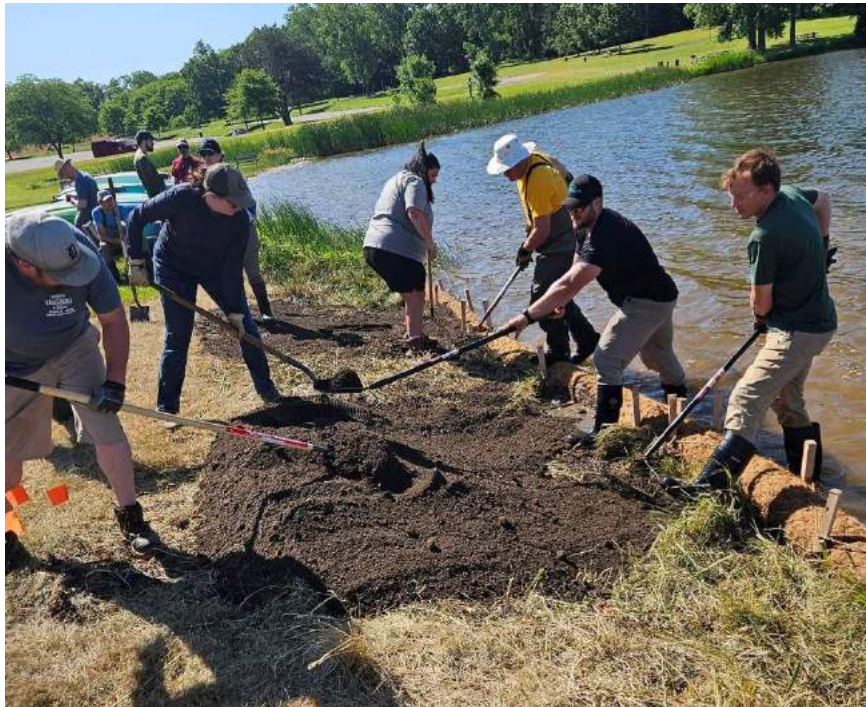
Figure 1: Natural Resources staff and class participants install natural shoreline at Stony Creek Metropark. Natural shorelines help prevent erosion through stabilization with native plants while also providing habitat for wildlife.
