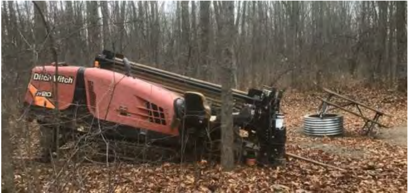
Pontiac Lake Recreation Area Campground Electrical Replacement Project
