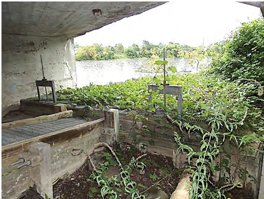
Photograph 16 – Fish ladder as it outlets downstream of the bridge.
