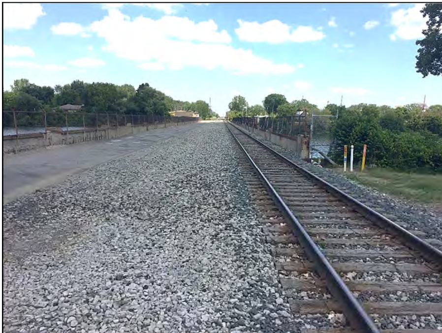
Photograph 2 – Abutment crest viewed from right
