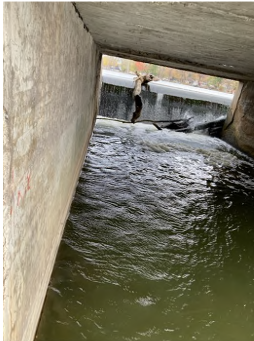
Photo #10: Principal Spillway Abutment Right Wall.
