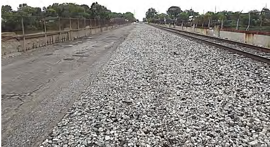
Photograph 2 – Embankment crest viewed from right.
