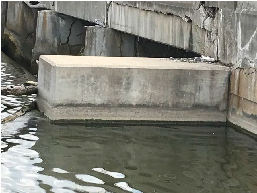
Photograph 9 – Right upstream abutment wall
