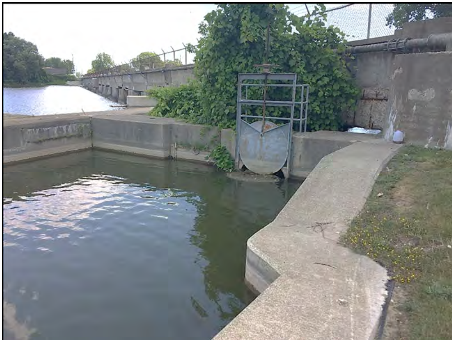
Photograph 16 – Abandoned lock gates Note that the right sluice gate feeds the fish ladder
