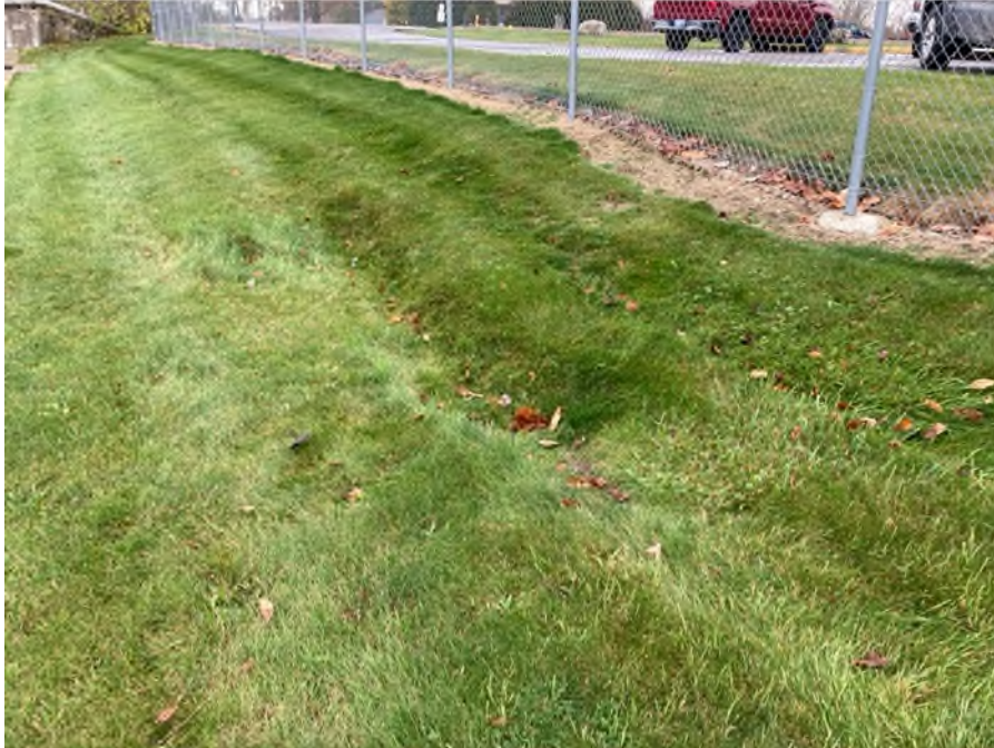
Photo #31: Embankment Upstream Slope. Issue: Depression, Action: Maintenance.
