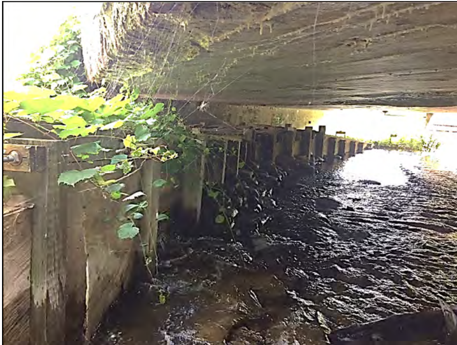
Photograph 18 – Wooden fish ladder viewed from upstream
