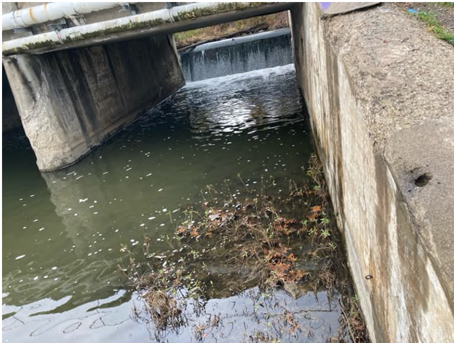
Photo #8: Principal Spillway Abutment Left Wall.
