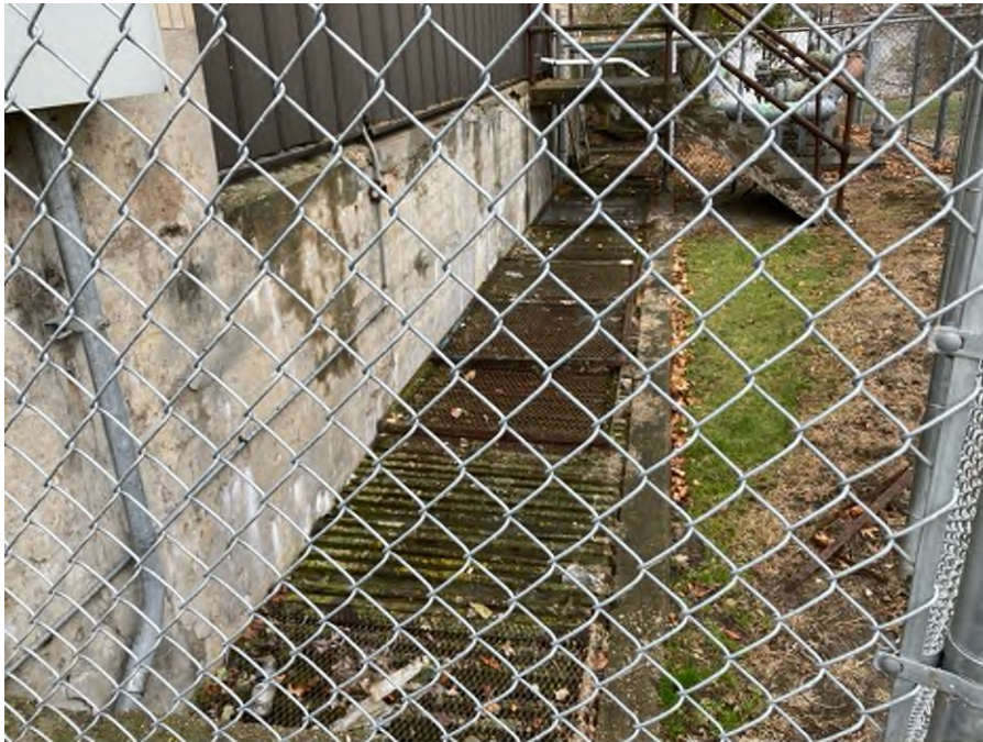
Photo #13: Auxiliary Spillway Left Chute.
