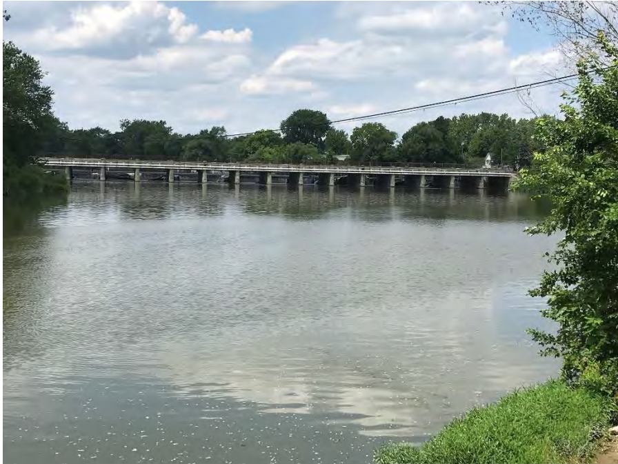
Photograph 7 – Principal spillway viewed from downstream
