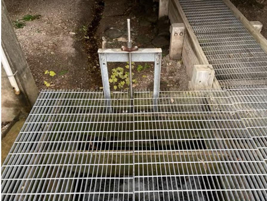
Photo #23: Fish Ladder Outlet 2 Gate.
