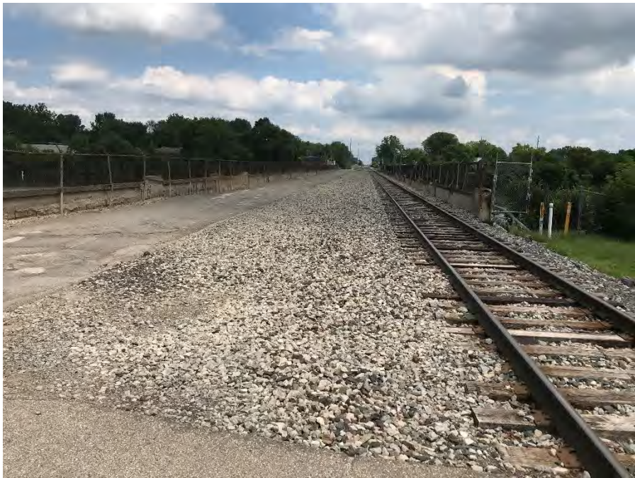
Photograph 2 – Abutment crest viewed from right
