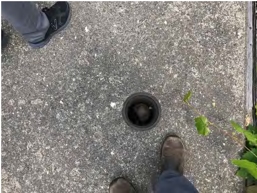
Photograph 20 – Left gate operator
