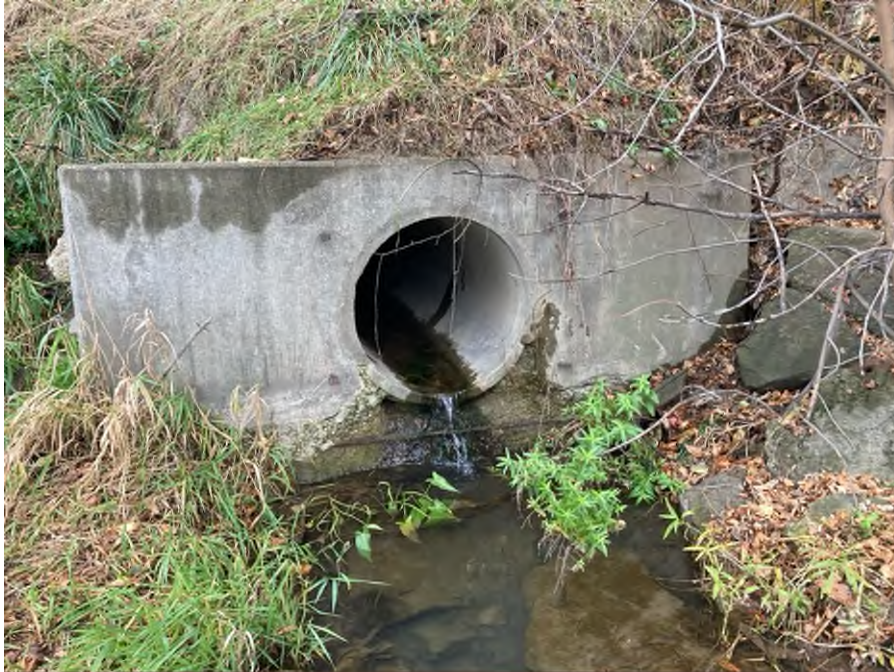
Photo #35: Embankment Downstream Slope. Drainage pipe for roads.
