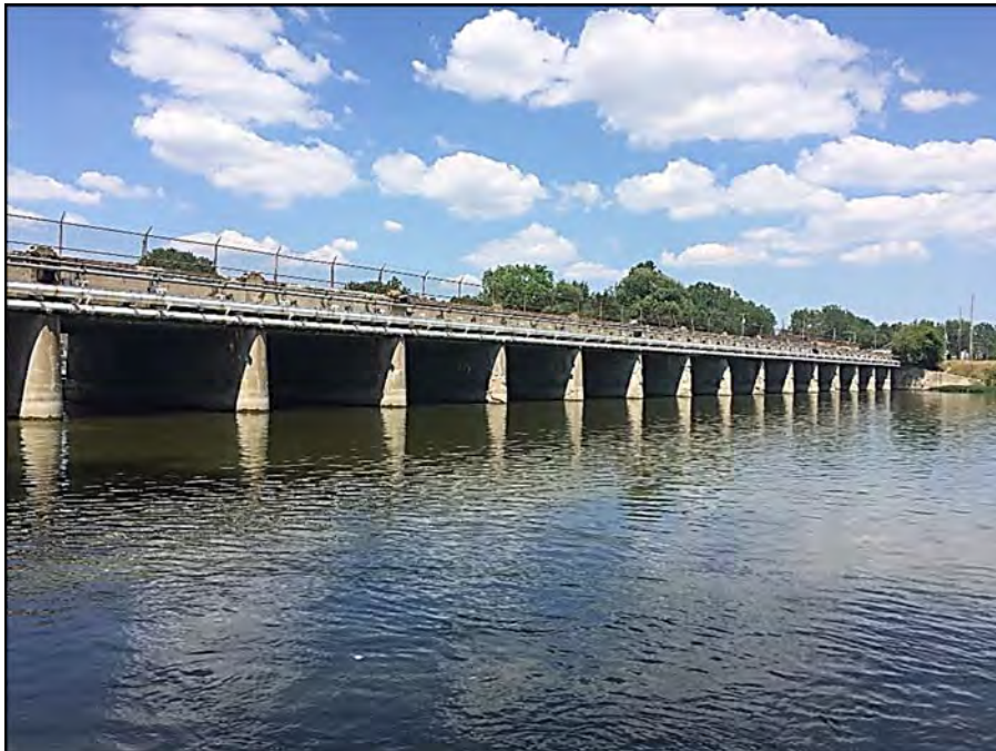
Photograph 12 – Downstream bridge viewed from right
