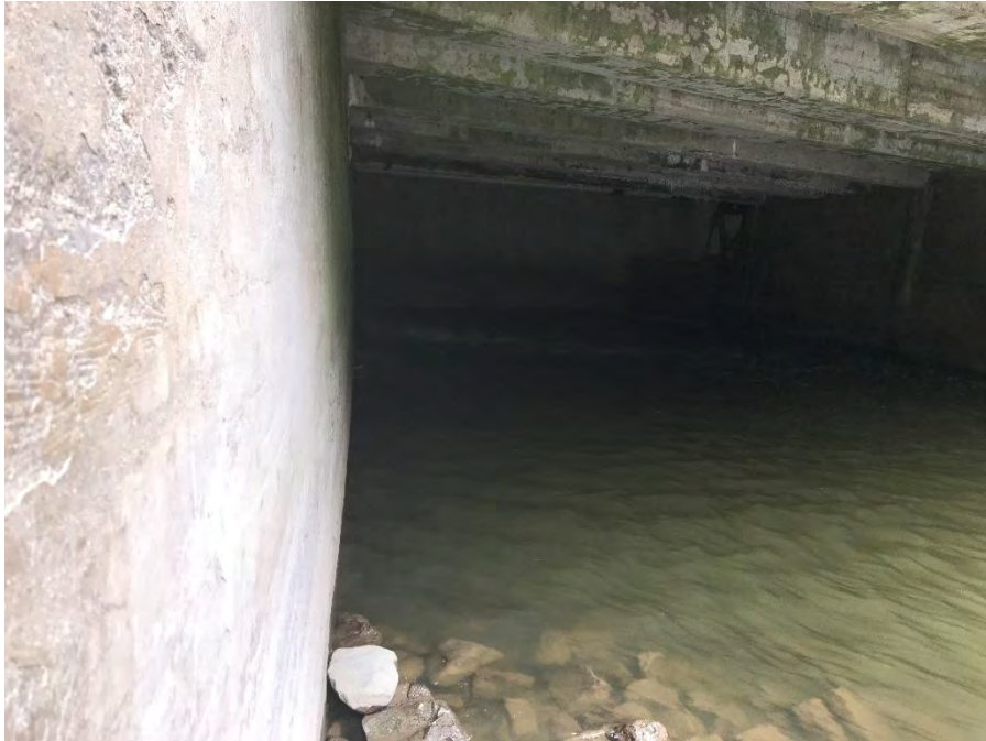
Photograph 25 – Powerhouse outlet viewed from downstream Note the flow from the right
