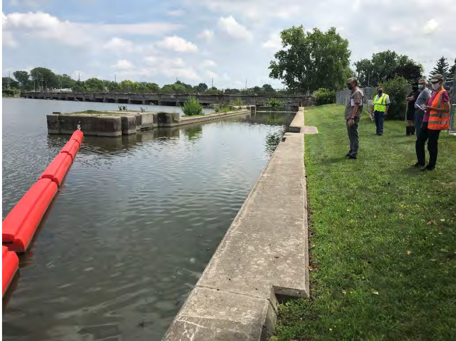
Photograph 16 – Right abutment wall of abandoned lock
