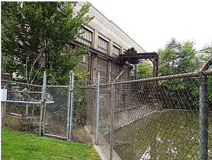
Photograph 18 – Abandoned powerhouse (now Flat Rock Steel) viewed from left.
