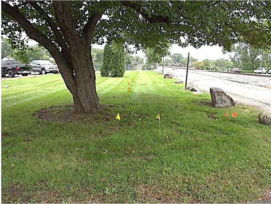
Photograph 1 – Upstream face of right embankment viewed from right.
