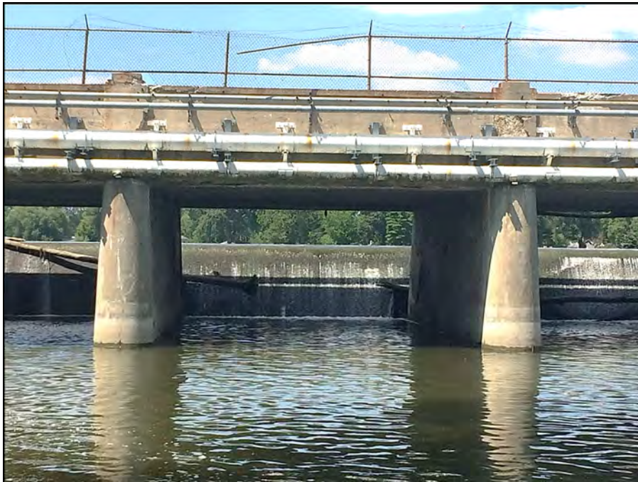
Photograph 14 – Typical spillway bay viewed from downstream
