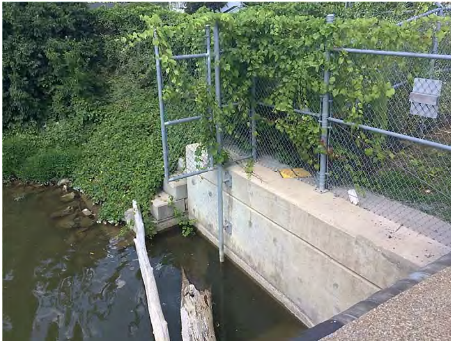
Photograph 8 – Upstream left spillway abutment wall
