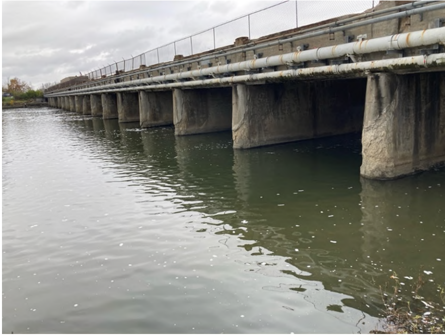
Photo #1: Principal Spillway Downstream.
