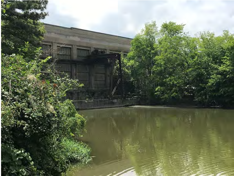
Photograph 23 – Former powerhouse inlet viewed from upstream
