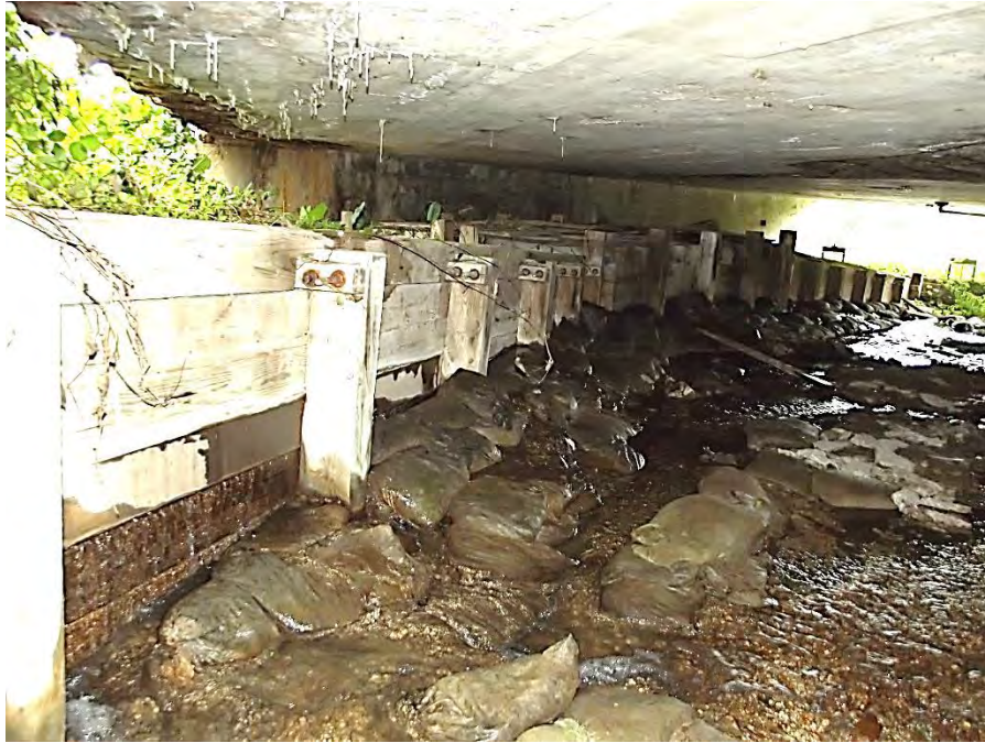
Photograph 15 – Fish ladder as it passes under bridge downstream of dam.
