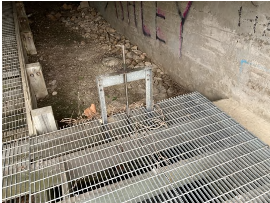
Photo #21: Fish Ladder Outlet 1 Gate.
