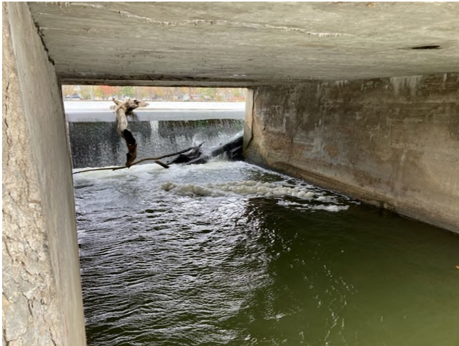
Photo #7: Principal Spillway Weir Wall.
