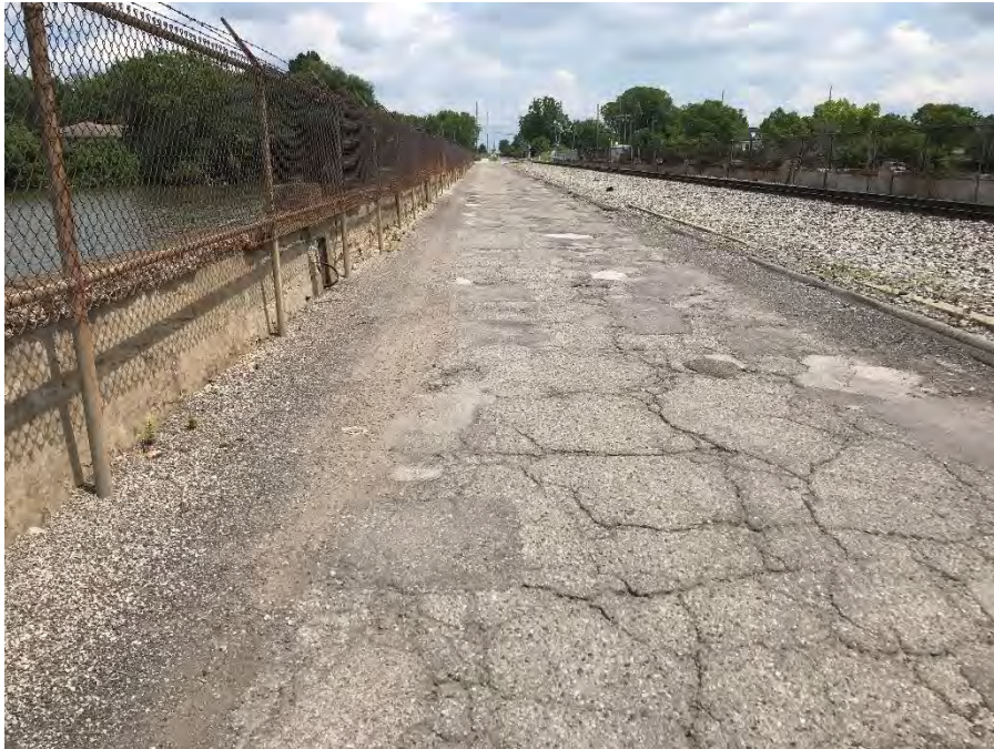
Photograph 5 – Left abutment crest viewed from left
