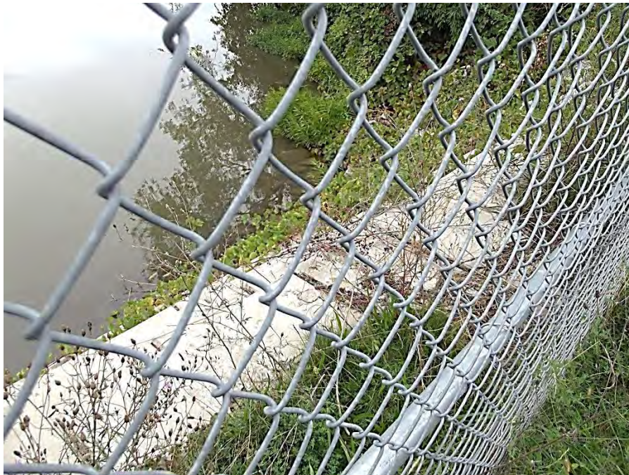
Photograph 4 – Upstream face of left embankment viewed from left.
