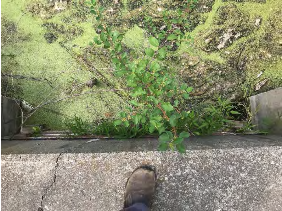
Photograph 19 – Left lock gate
