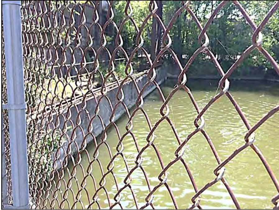
Photograph 19 – Powerhouse inlet viewed from left
