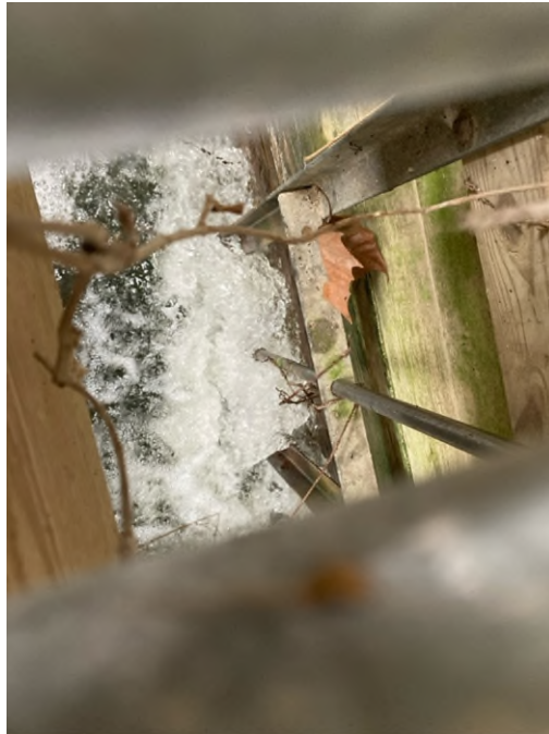
Photo #20: Fish Ladder Outlet 1 Gate.
