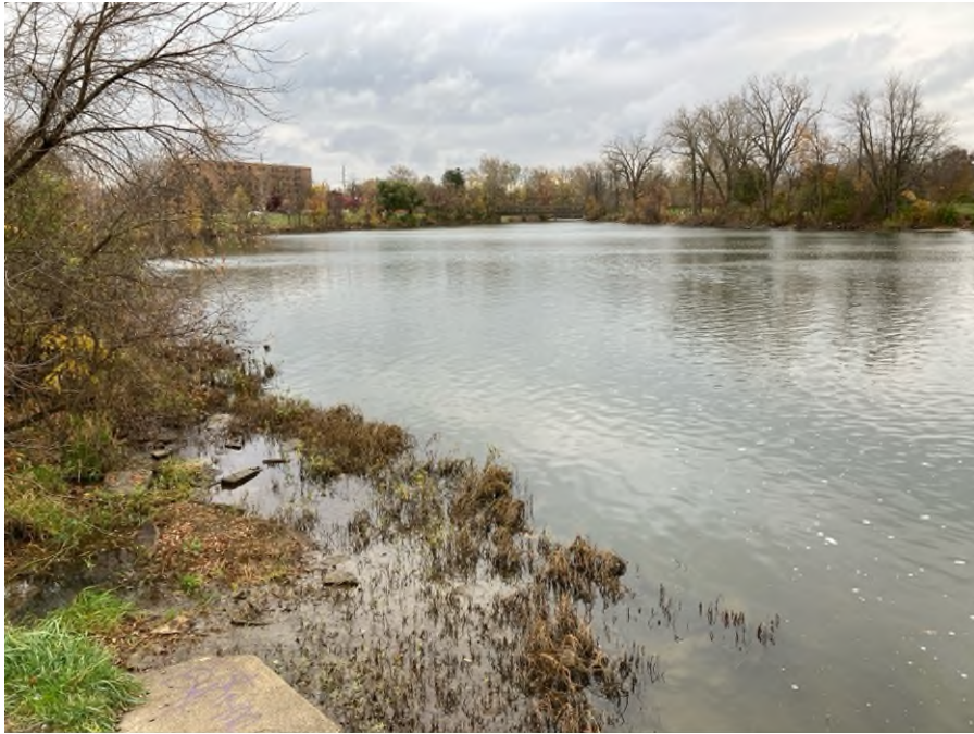
Photo #2: Principal Spillway Downstream.
