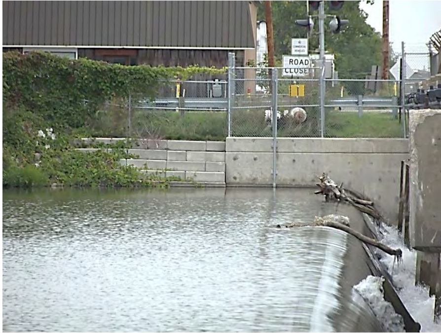
Photograph 9 – Upstream left principal spillway abutment wall viewed from right.
