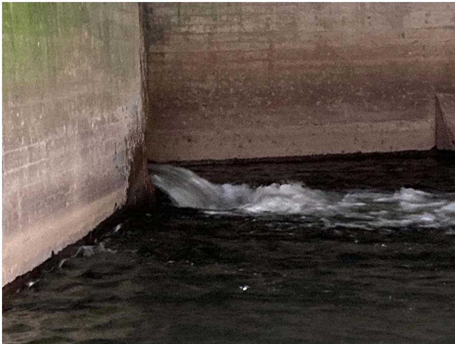
Photo #14: Auxiliary Spillway Right Chute Outlet.
