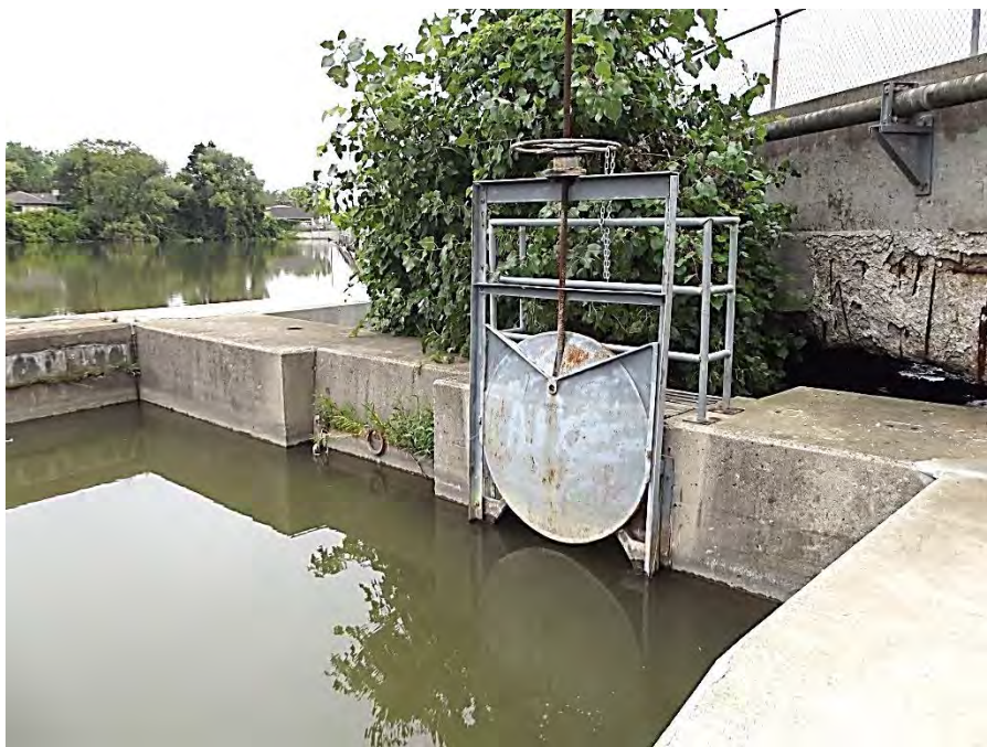
Photograph 14 – Gate system for abandoned locks. Note the raised gate now provides water for a downstream fish ladder.
