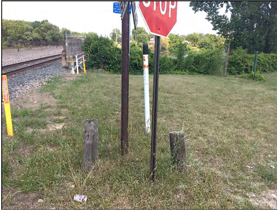
Photograph 3 – Downstream face of right abutment viewed from right
