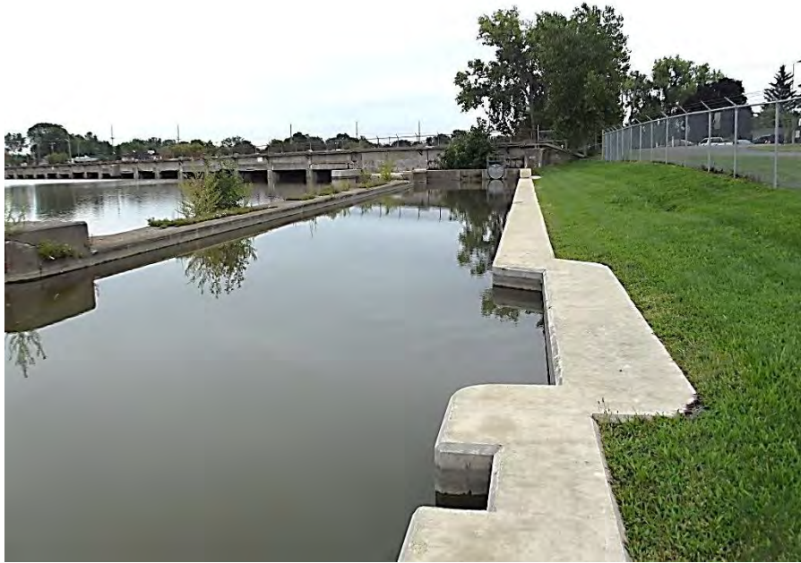
Photograph 7 – Upstream right principal spillway abutment wall viewed from upstream.
