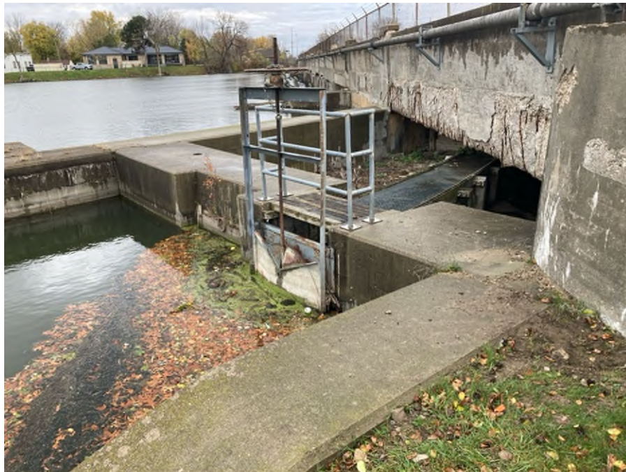
Photo #26: Fish Ladder Chute Inlet.
