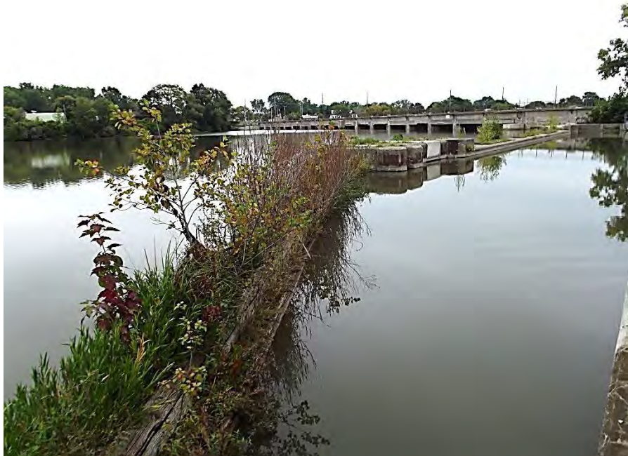
Photograph 11 – Inlet to abandoned lock system viewed from upstream. Note the overgrowth of vegetation at the log boom.
