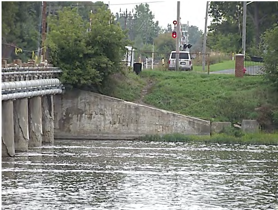
Photograph 10 – Downstream left principal spillway abutment wall viewed from right.
