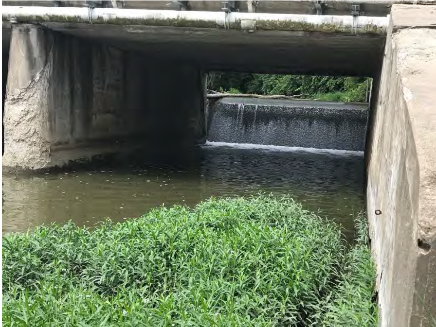
Photograph 13 – Typical spillway bay
