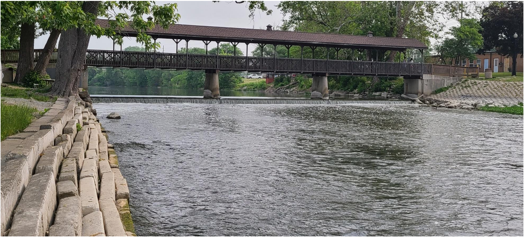
Figure 9. Looking Upstream Towards Huroc Dam and Pedestrian Bridge
