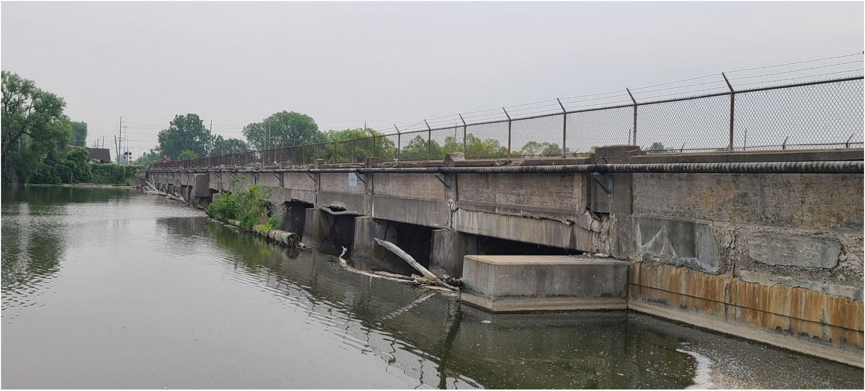
Figure 5. Looking Downstream Towards Flat Rock Dam and Railroad Bridge
