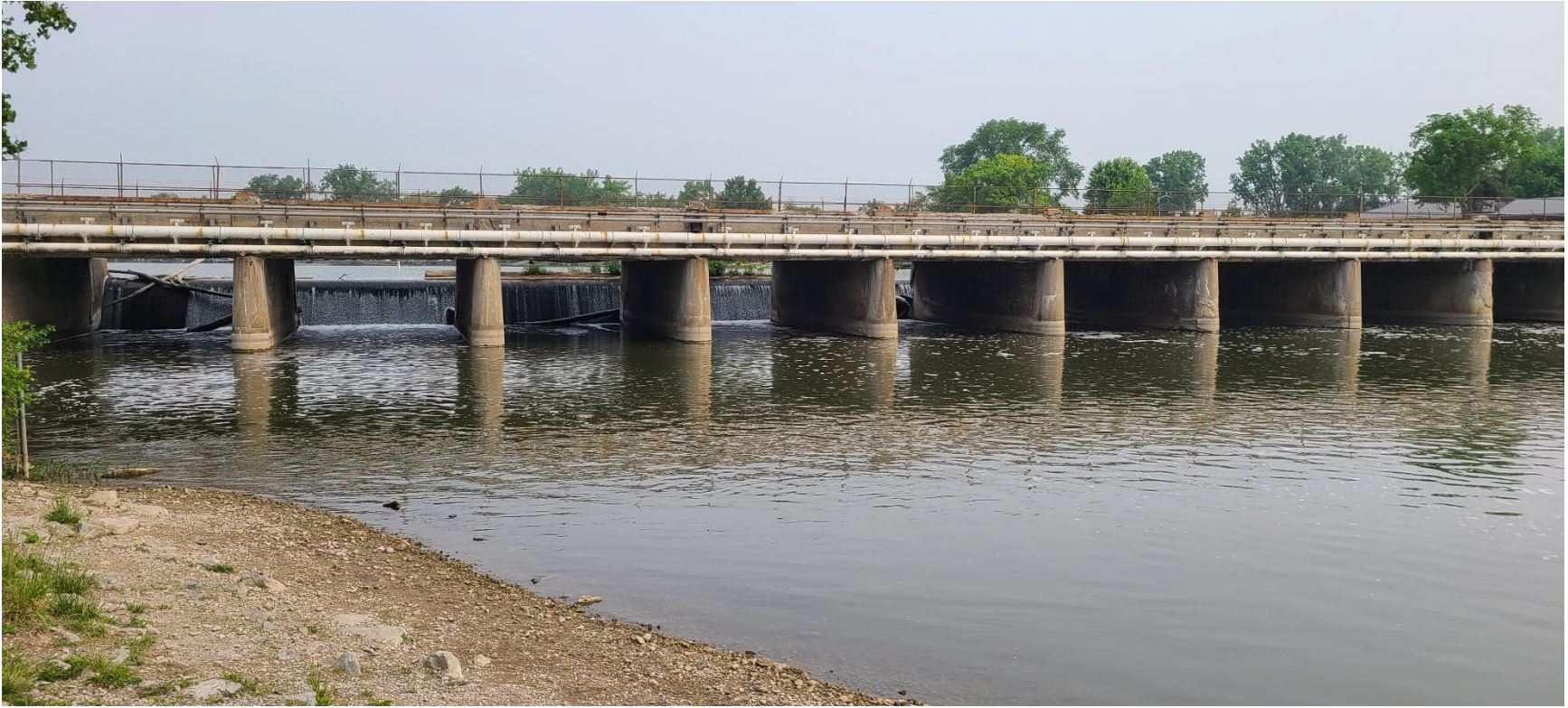
Figure 6. Looking Upstream Towards Flat Rock Dam and Railroad Bridge
