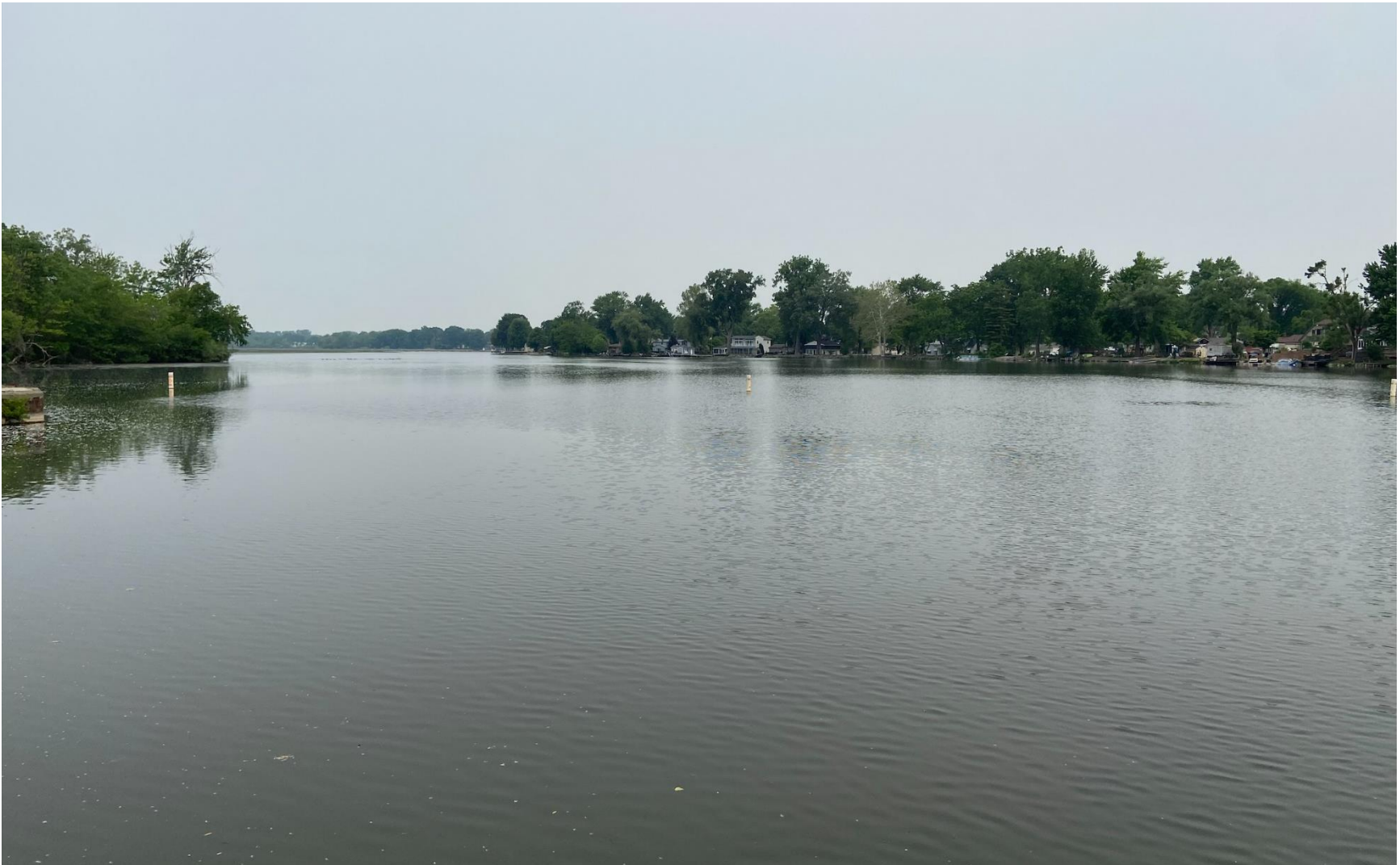
Figure 4. Looking Upstream from Flat Rock Dam at Forested Floodplain
