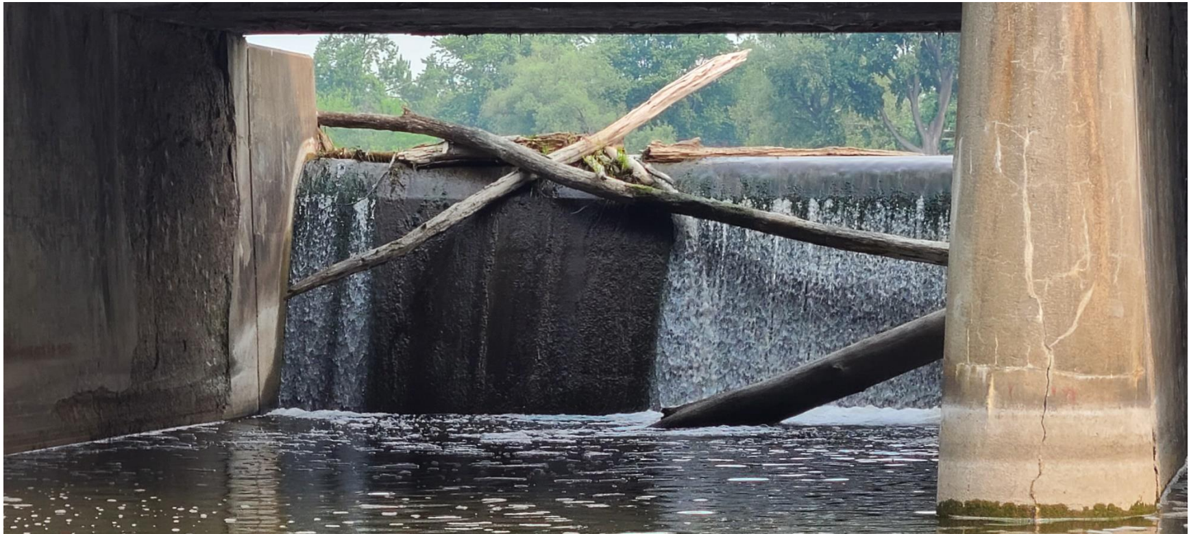
Figure 7. Looking Upstream Towards Flat Rock Dam and Railroad Bridge Zoomed In
