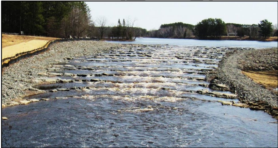
Figure 14 : Looking Upstream at a Completed Rock-Arch Rapids Project Designed by Dr. Aadland on the Willow River of Minnesota
