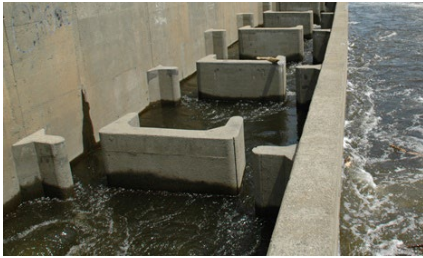
Figure 10: An Example of a Vertical Slot Fishway
