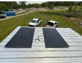
Staff installed two solar panels and four lithium iron phosphate batteries, and one charger/inverter to be installed at Stony Creek, Eastwood Beach, paddle shack.
