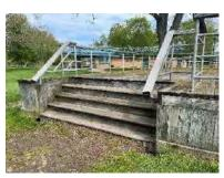
The existing boardwalk decking, handrails, lighting and other appurtenances will be removed and replaced with new finishes to create a rehabilitated elevated boardwalk system
